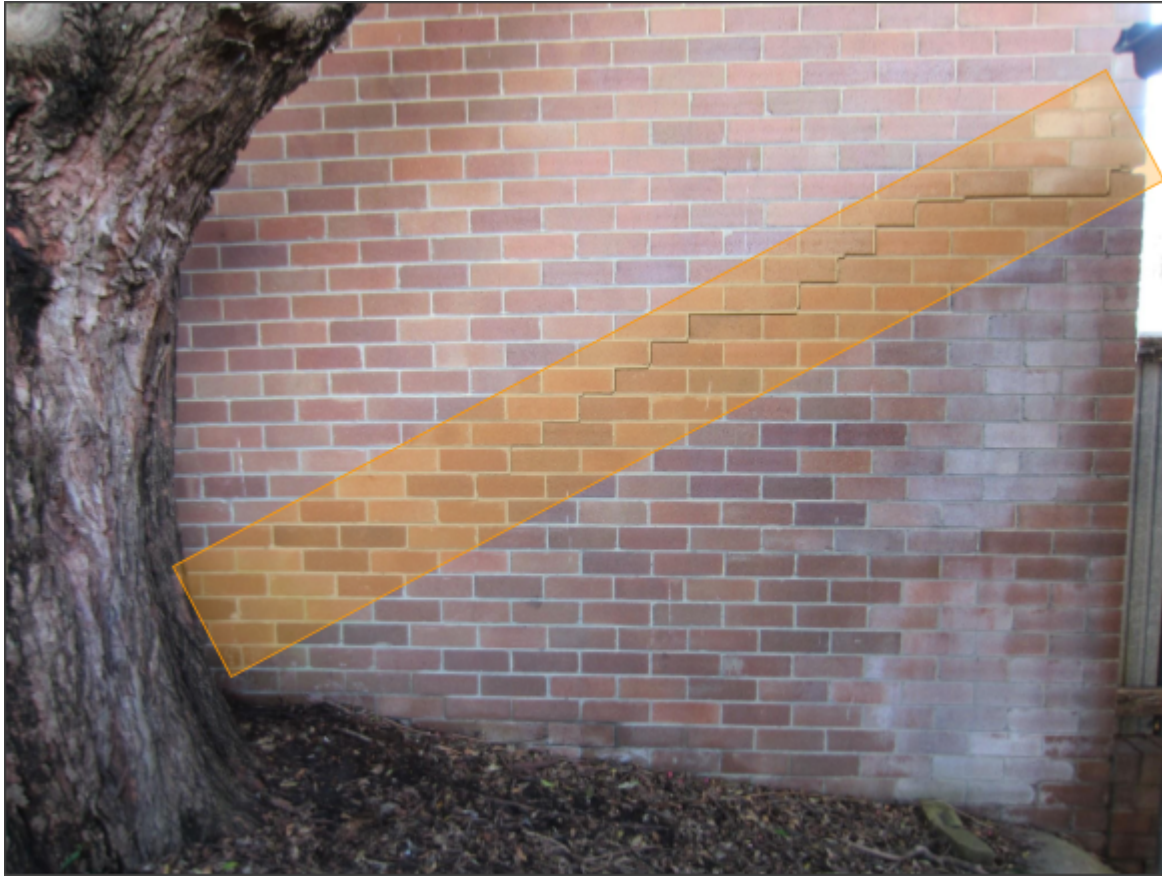
Photo D: Highlighting the extent of the crack in the wall. Tree viewed from south.
